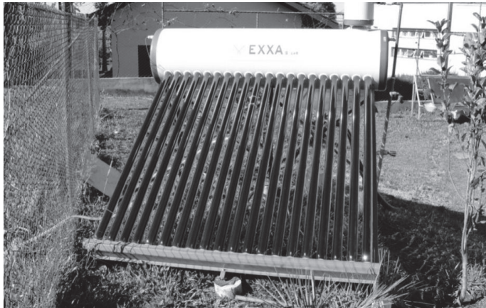
Figure 1. Solar collector with vacuum tubes type all-glass.
